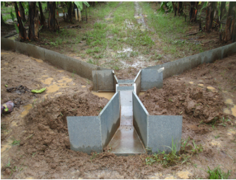
Flumes capture surface run-off and help researchers assess the level of sediment and nutrient movement after rainfall.
