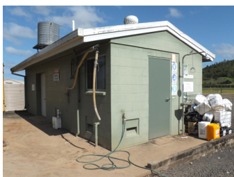
Chemicals should be stored in a specifically-designed and designated area.
