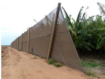
Constructed wind breaks are used to prevent wind erosion in Carnarvon.
