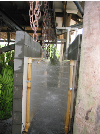
Review the water use and where efficiencies can be introduced.
