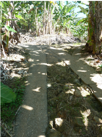
Concrete roadways provide all weather access in steeper areas, for example on the subtropics east coast.
